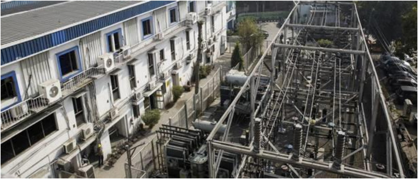
View of TATA Power DDL, Power House, Rohini, New Delhi from the top
